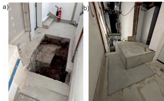
Figure 2: Basement for a beam transport vacuum chamber. a ) exposed problematic area. b) newly cast base.
